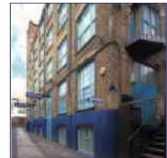
Imperial Works Kentish Town, London NW5 Characterful offices with residential conversion potential. Acquisition – June 2014
